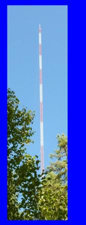
Park Falls WLEF tower (US-PFa) EC fluxes at 30, 122, 396 m NOAA tall tower greenhouse gas site COSMOS soil moisture TCCON column GHG
